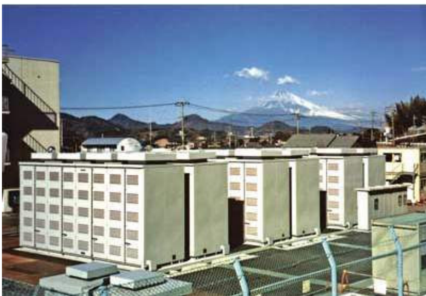
The NAS battery installation at Tokyo Electric Power Co.'s Ohito Substation is rated at 6 MW/48 MWh
